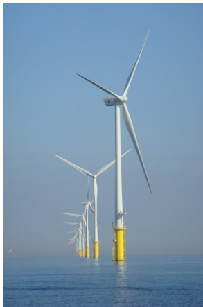
Wind farm Internal & External Inspection
